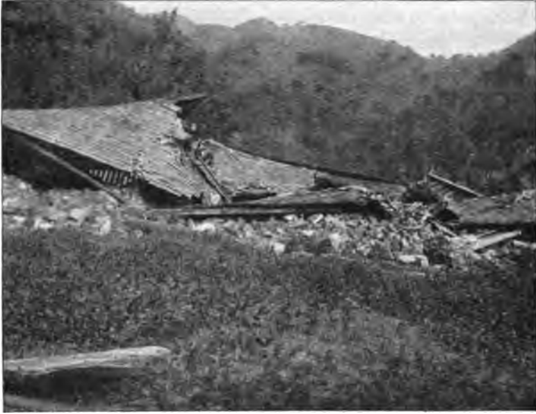
FIG. 3.—THE GARDENS HOUSE, GORDON TOWN.
