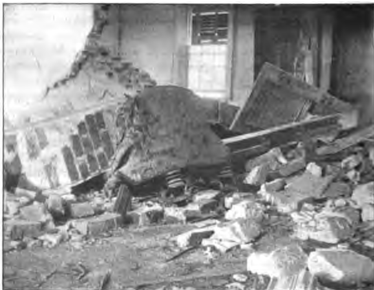
FIG. 2.—FIRST-FLOOR DRAWING-ROOM OF HOUSE IN EAST STREET, KINGSTON.
